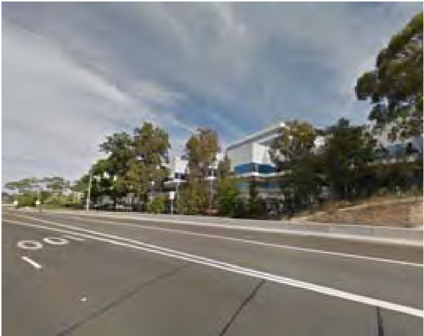
View 05 M2 Looking South toward Site
