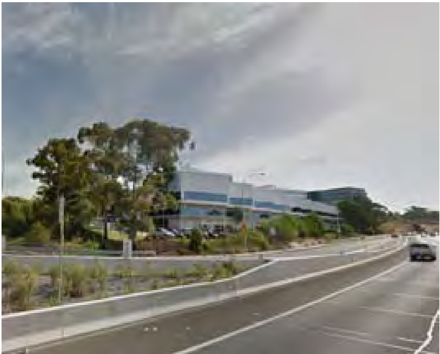
View 04 M2 Motorway looking North toward Site
